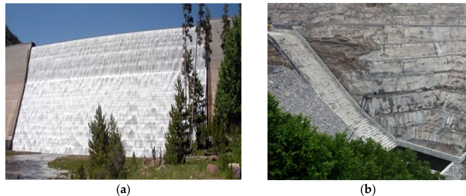
Figure 1. Stepped spillways with an abrupt slope reduction (a) Upper Stillwater dam, USA ( http://www.usbr.gov , last accessed date: 15 November 2013); (b) Siah-Bishe lower dam, Iran ( http://www.iwpc.ir , last accessed date: 21 February 2016).
