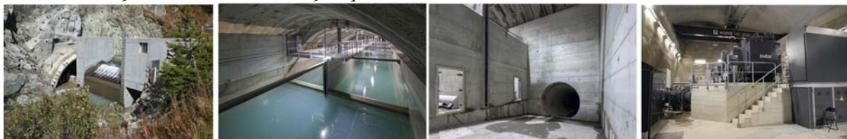
Figure 1 Picture of the intake, the silting chamber, the forebay tank with the inlet of the headrace tunnel and the machinery cavern of KWGO SHP, source: FMV
