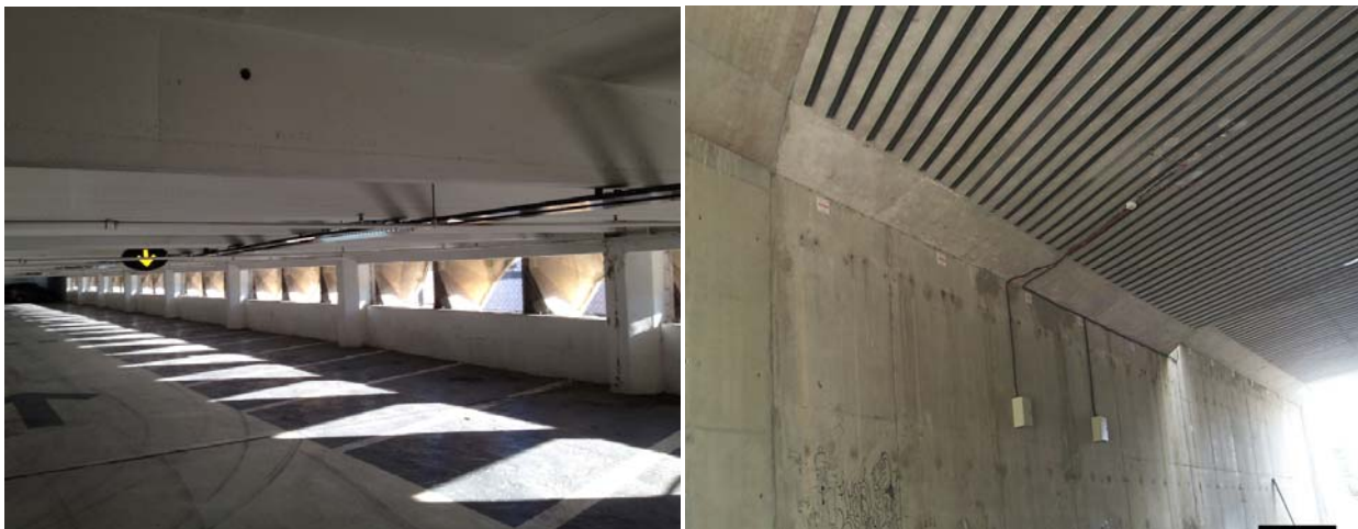
(a) Beams of Parking strengthened by EBFRRP
