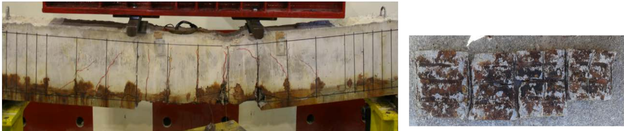
Figure 5: Flexural crack pattern of corroded beam RC-COR1 after testing to failure.
