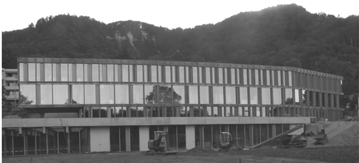
Figure 2: College building Zurich Falletsche: filigree vertical CFRP prestressed HPSCC façade columns
