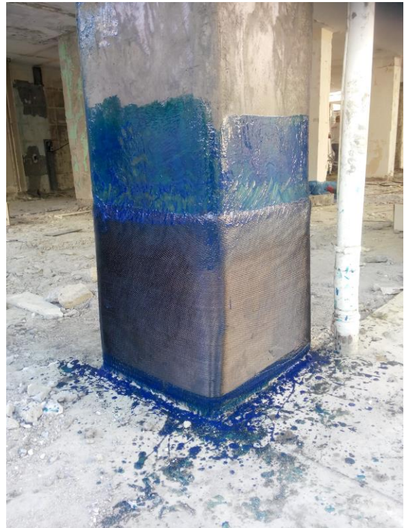
Fig.8 – CFRP Application on Corner Columns
