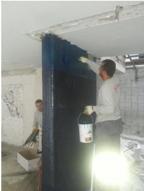
Fig.7 – CFRP Application on Shear Walls
