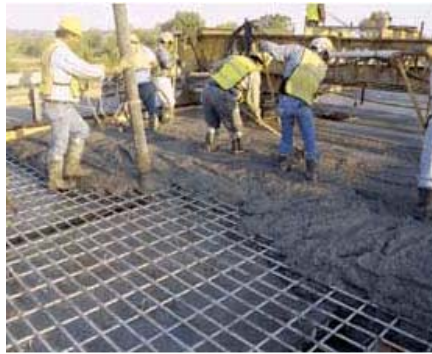
Fig. 2 Bridge deck reinforcement with GFRP.
