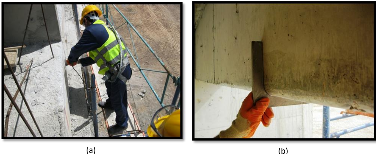
Figure 2: Concrete surface preparation and corner rounding proses
