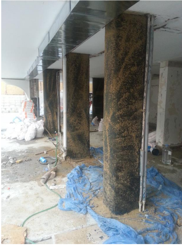
Fig.9 – Sand Cover for Better Plastering
