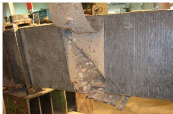
(i) Full wrapping with continuous FRP sheets
