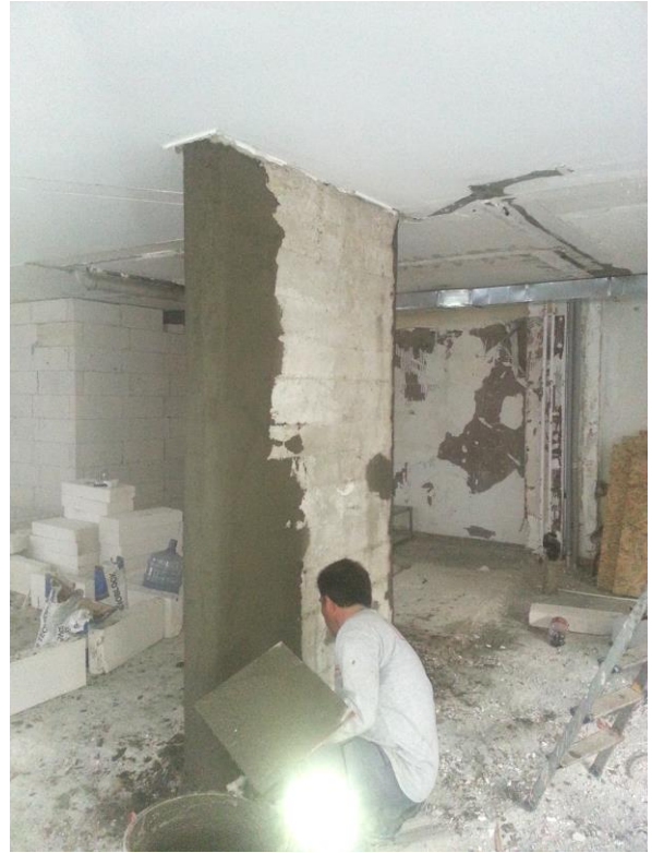
Fig.6 – Restoring the Original Cross-Section
