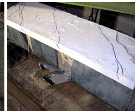
(iii) U-jacketing with FRP sheets
