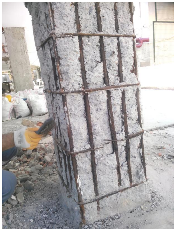
Fig.4 – Cleaning on Corner Column
