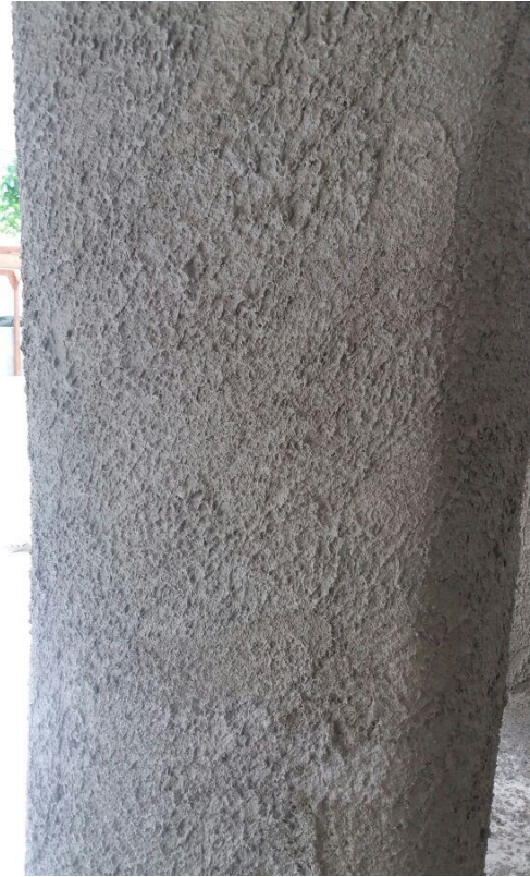
Fig.10 – Plastering Against Fire
