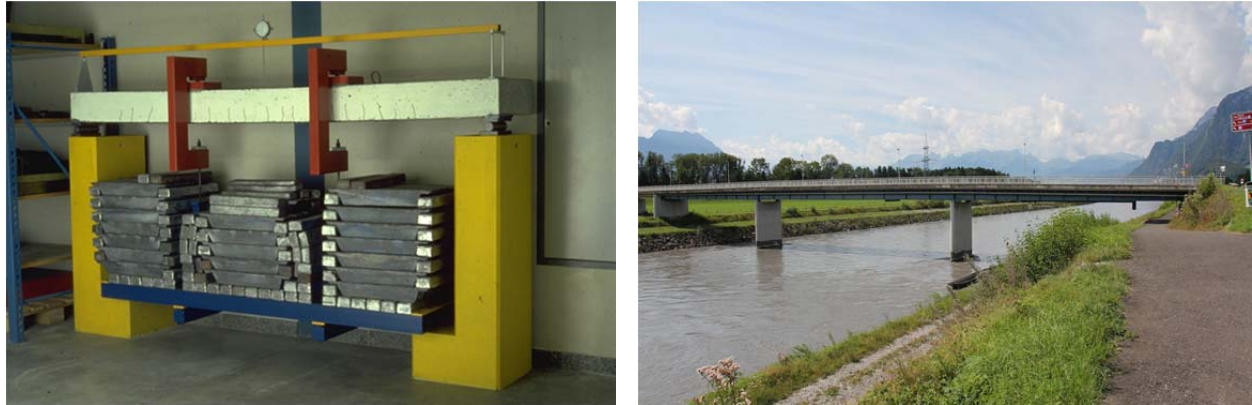
Figure 5: Left: long-term test at Empa since 1970, the reinforced concrete beam was strengthened with a steel plate by using an epoxy adhesive. Right: Rhine bridge between Switzerland and Austria, which was strengthened with unstressed CFRP strips in the year 1996.
