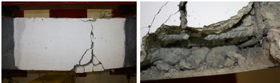
Figure 2. Steel failure of beam REX20-H at 990,147 fatigue cycles
