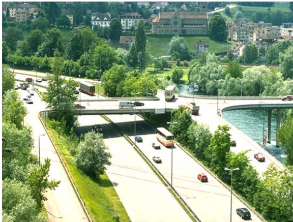
Ibach bridge in Switzerland, first application of CFRP strips on a civil structure in 1991
