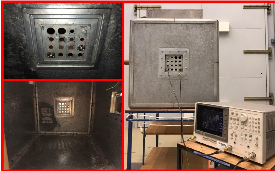
Figure 12. Experimental setup including the location of the antennas, the interior side of the cavity considered as the transformer tank, and the Vector Network Analyzer (VNA) that is used to measure the scattering parameters.
