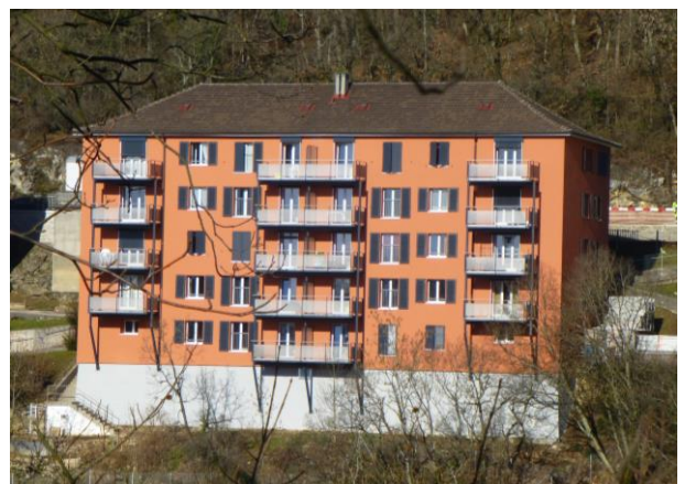
Figure 6 Orée 50: Renovation and insulation of facades, replacement and enlargement of balconies (Archetype 3, Renovation type II). Pictures from architect.
