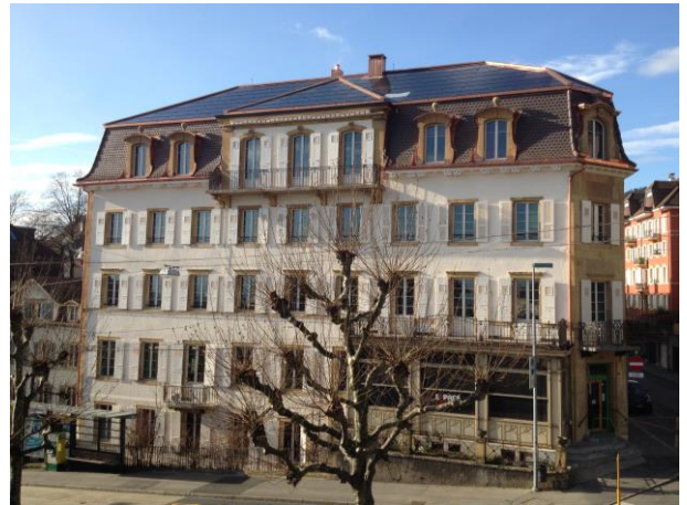
Figure 4 Louis-Favre 1: Roof replacement, installation of 171 m 2 of integrated photovoltaic cells for a production of about 27.7 kWp (Archetype 1, Renovation type I). Pictures from Pro Natura Neuchâtel (left) and from the architect (right).
