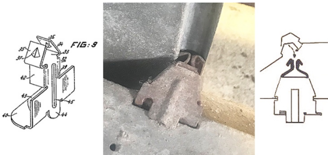
Figure 5. Clip for cladding: Patent FR1079026A, published: 25.11.1954 (Jungo). Photo of clip in Fribourg, 2022 (Transform). Clip detail, 1958 (Archives Ville de Fribourg)
