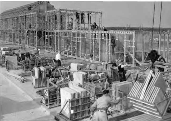
Figure 2. POLYNORM building site, Eindhoven, 1951 (Philipps Company Archive).
