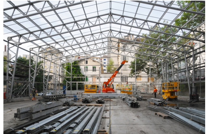
Figure 9. Dismantling POLYNORM hall in Fribourg, 14.09.2022 (Transform).
