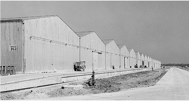
Figure 8. POLYNORM hall built by US Air Force, 1953, Châteauroux-La Martinerie, F (www.france-air-nato.net).
