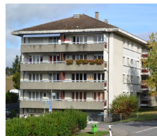
Figure 2. Typical post-WW2 building as Swiss suburban standalone (1972).
