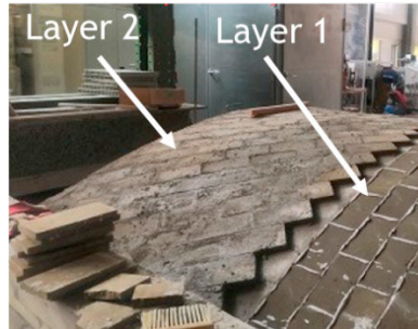
Fig. 2. A Catalan vault being built. Excavation earth bricks are used.
